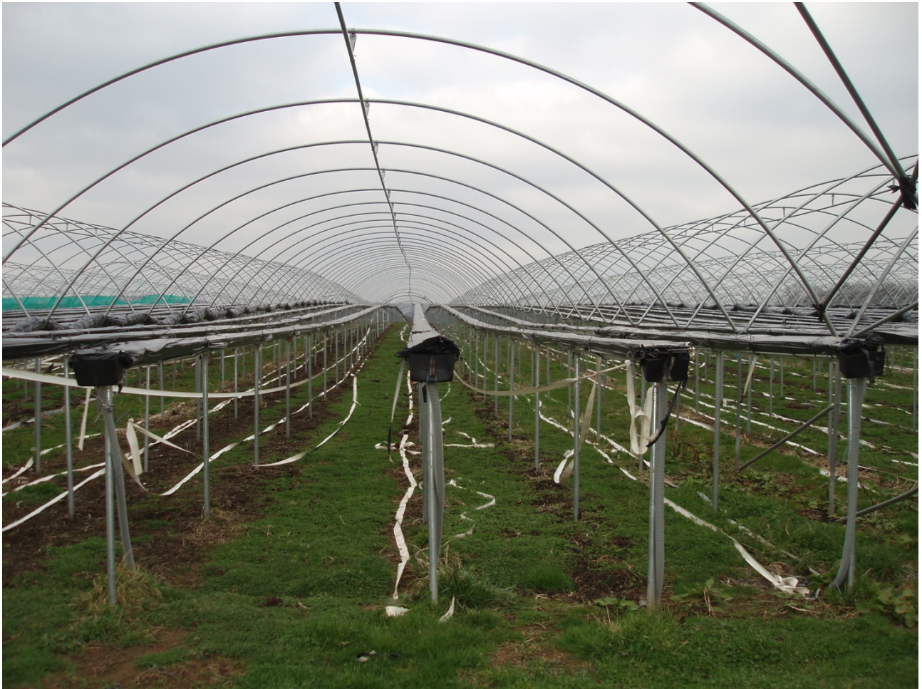
Figure 6: Table-top growing involves the precise fixing of 'legs' within the polytunnel structure to aid the effectiveness of trickle irrigation, but also necessitates permanent tunnels to justify the capital investment.
