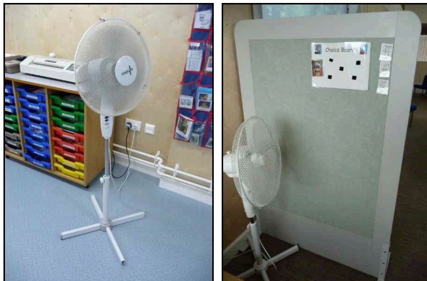
Figure 11.13: Free-standing fans in the new classrooms
