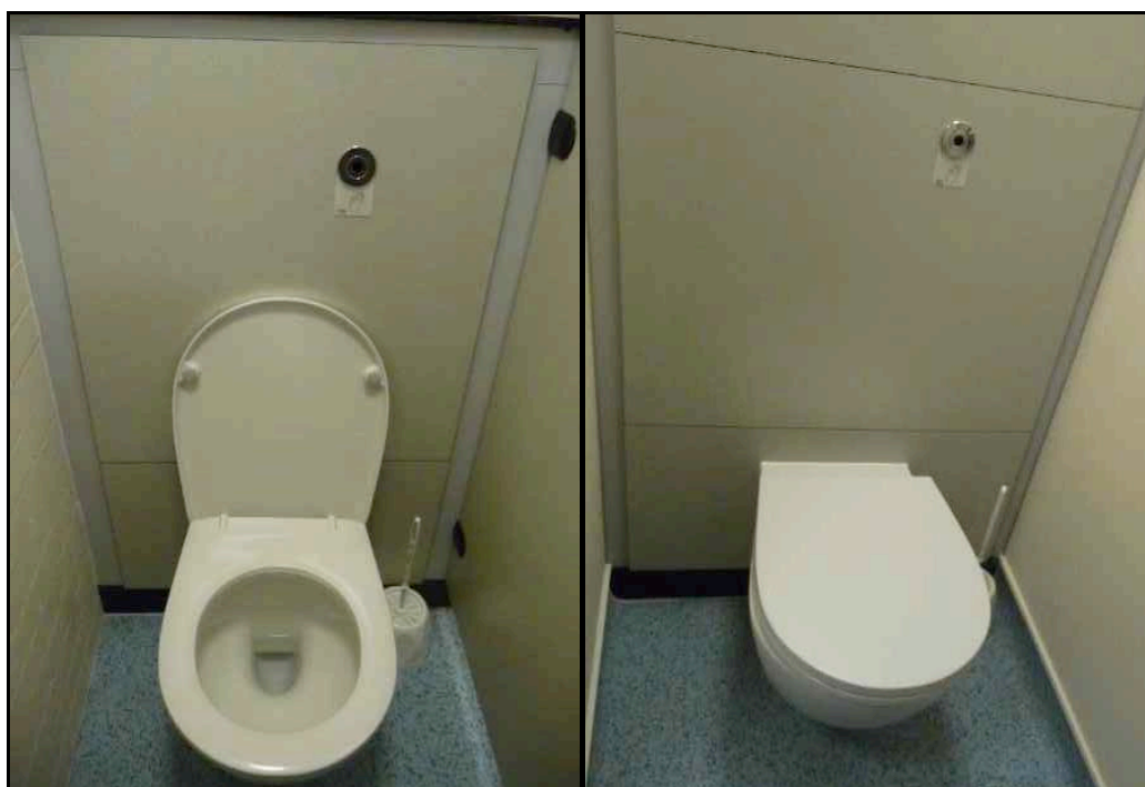
Figure 9.4: 'Boxed-in' toilets in the new school
