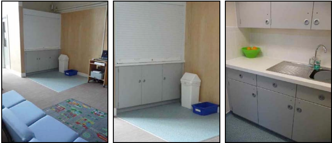
Figure 11.19: Kitchenette and kitchen areas within the new school, shown both with protective shutter up and down.
